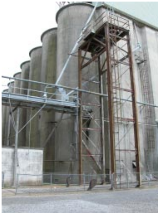
Concrete storage tanks at Beaumont Rice Mill.
