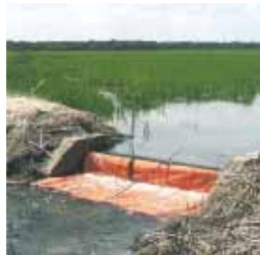
These pictures taken at L.G. Raun's farm in El Campo illustrate a cement 'water box' used to control water flow across levees. According to L.G., these improve water management by saving time and resources.
