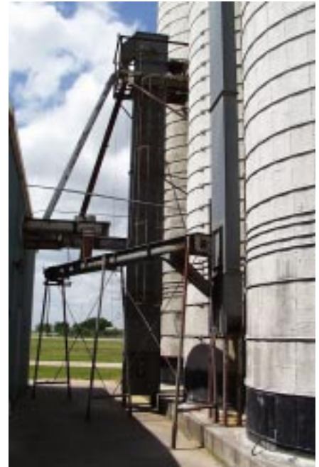
Commercial rice drying operations require intense monitoring of bin temperature, moisture and airflow.
